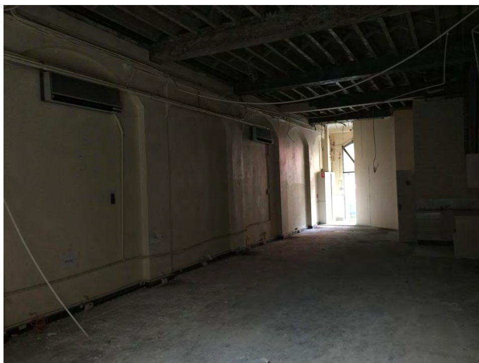
Figure 88 – Space G06 looking west. NBRSPartners, April 2015.
