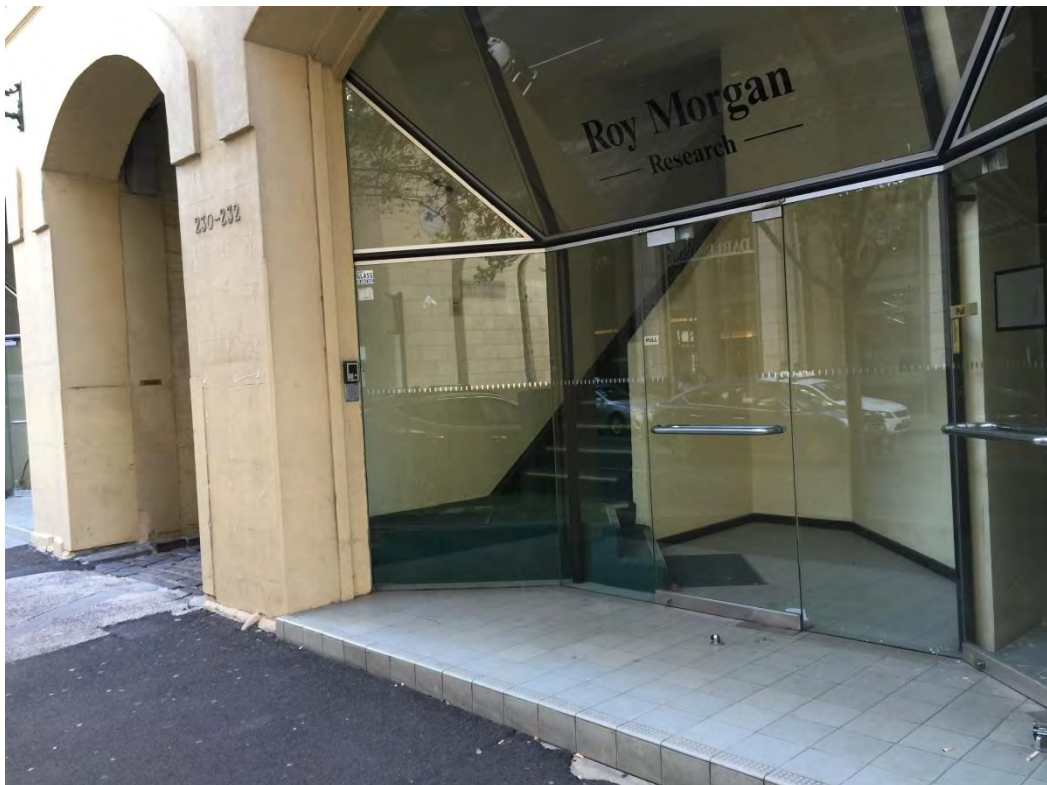
Figure 58 – Ground floor façade opening infill. NBRSPartners, April 2015.
