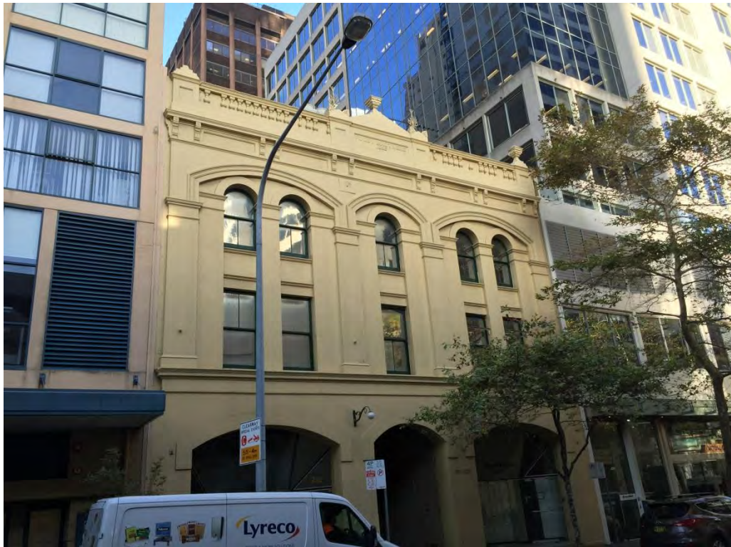
Figure 53 – Façade. NBRSPartners, April 2015.
