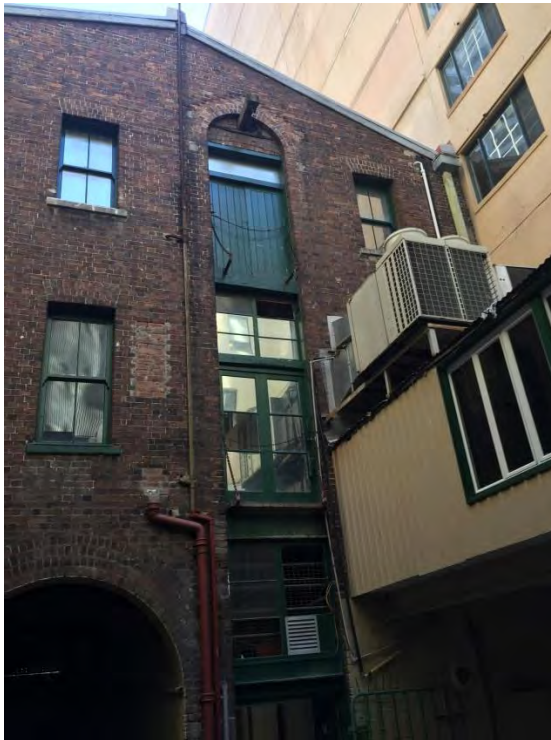
Figure 60 – Eastern elevation of warehouse. NBRSPartners, April 2015.
