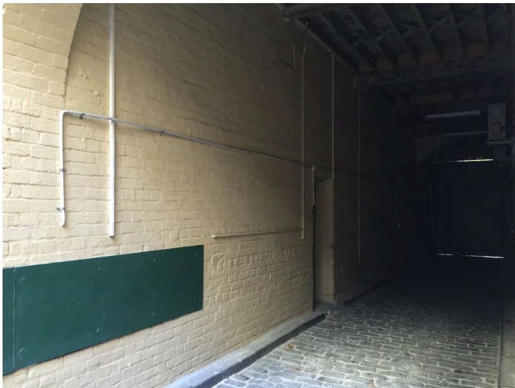
Figure 70 –Cartway (Y01) looking west. NBRSPartners, April 2015.
