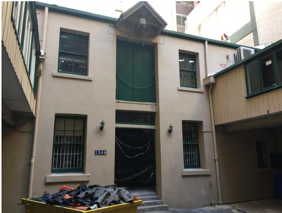
Figure 67 – Western elevation of rear warehouse from yard (Y02). NBRSPartners, April 2015.
