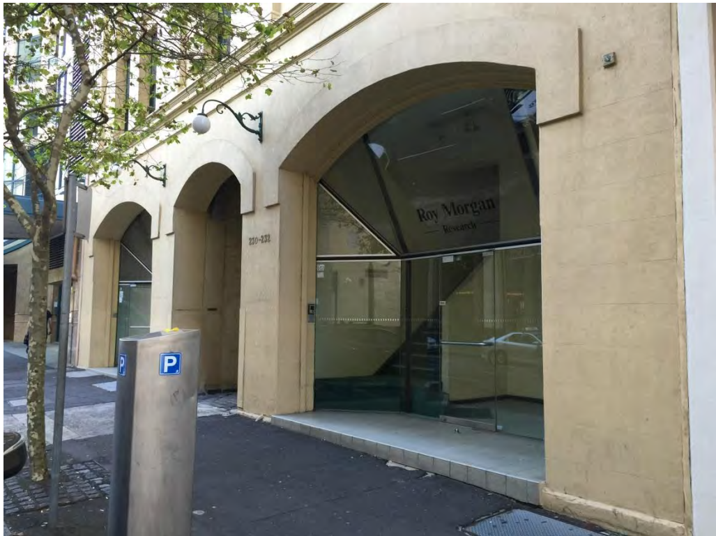
Figure 49 – Ground floor on Sussex Street. NBRSPartners, April 2015.
