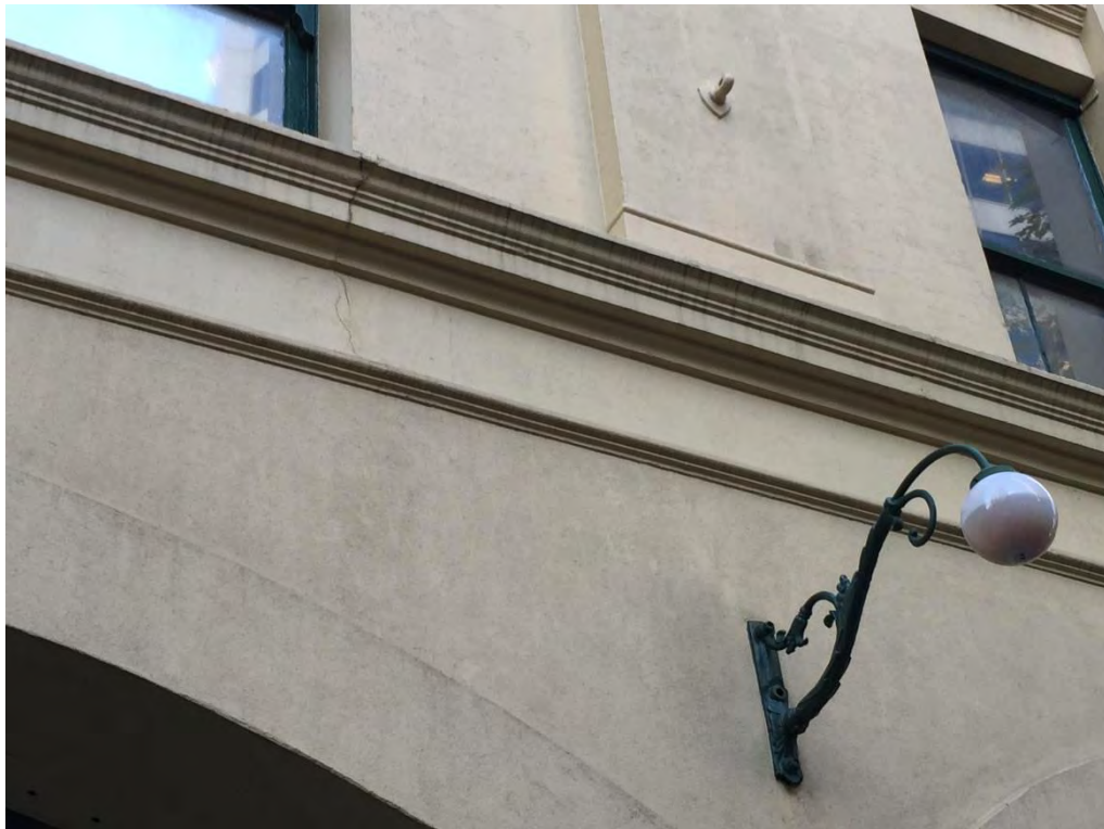
Figure 47 – ‘Period’ bracketed luminaires and original awning anchors. NBRSPartners, April 2015.
