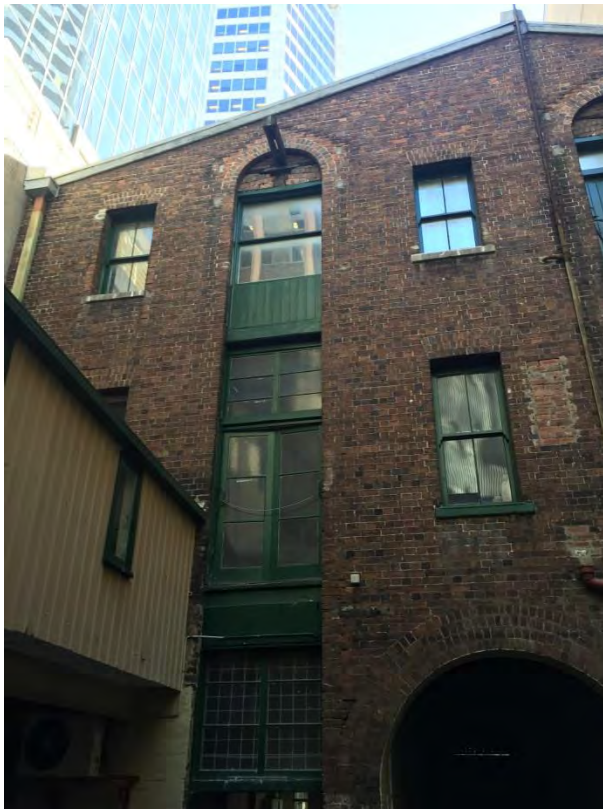
Figure 62 – Eastern elevation of warehouse. NBRSPartners, April 2015.
