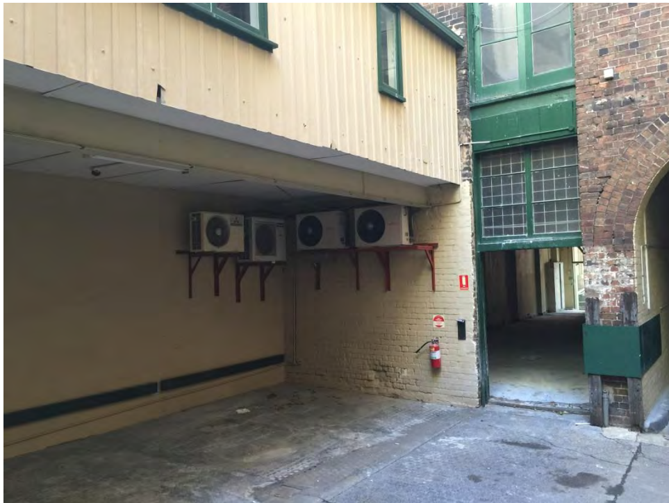
Figure 79 – Yard (Y02) looking southwest. NBRSPartners, April 2015.
