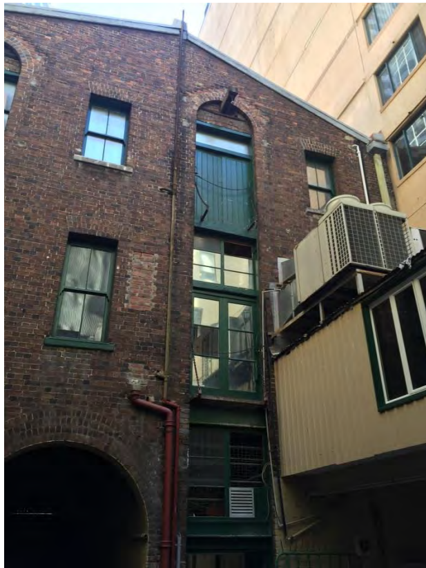
Figure 64 – Eastern elevation of warehouse. NBRSPartners, April 2015.
