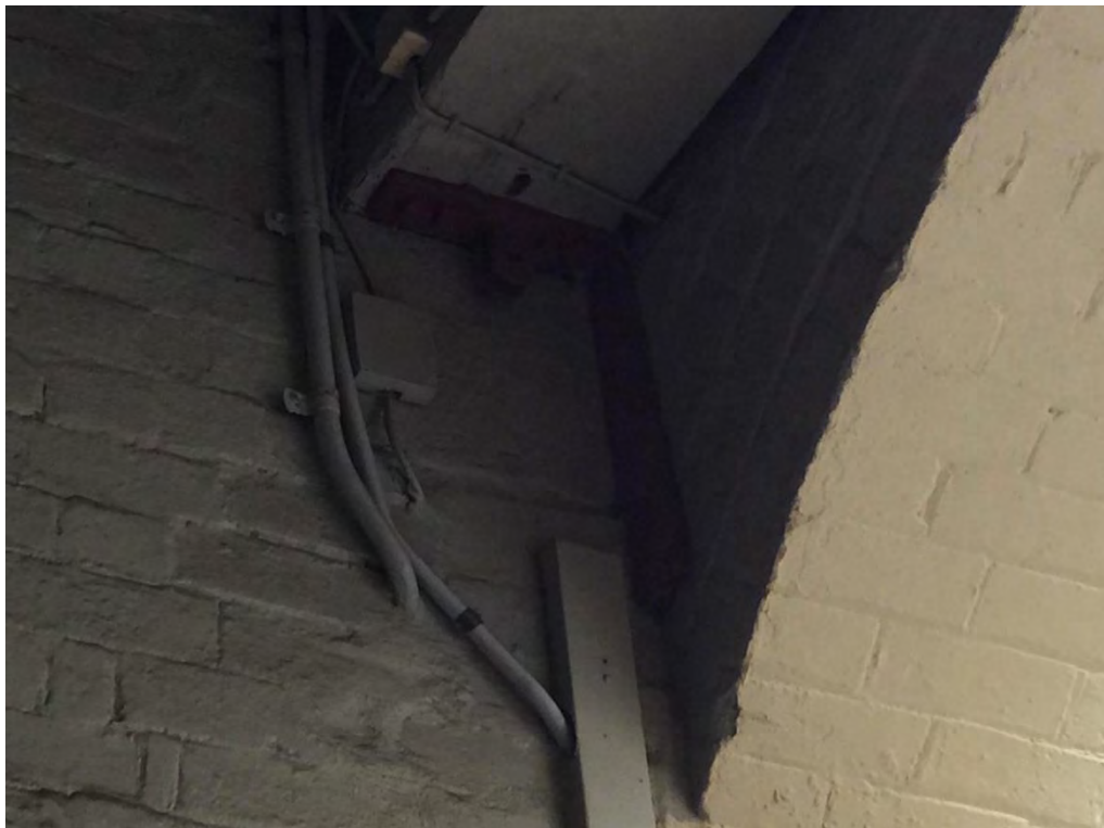
Figure 56 – Pivot brackets as evidence of original cartway gates. NBRSPartners, April 2015.
