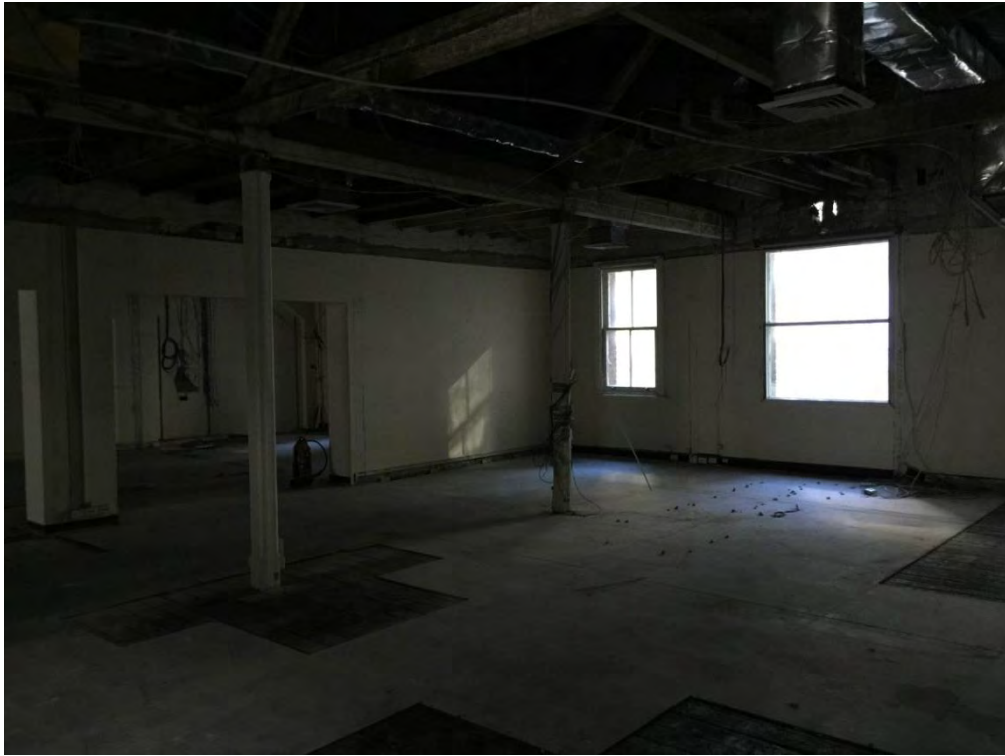
Figure 95 – Eastern section of space S02. NBRSPartners, April 2015.
