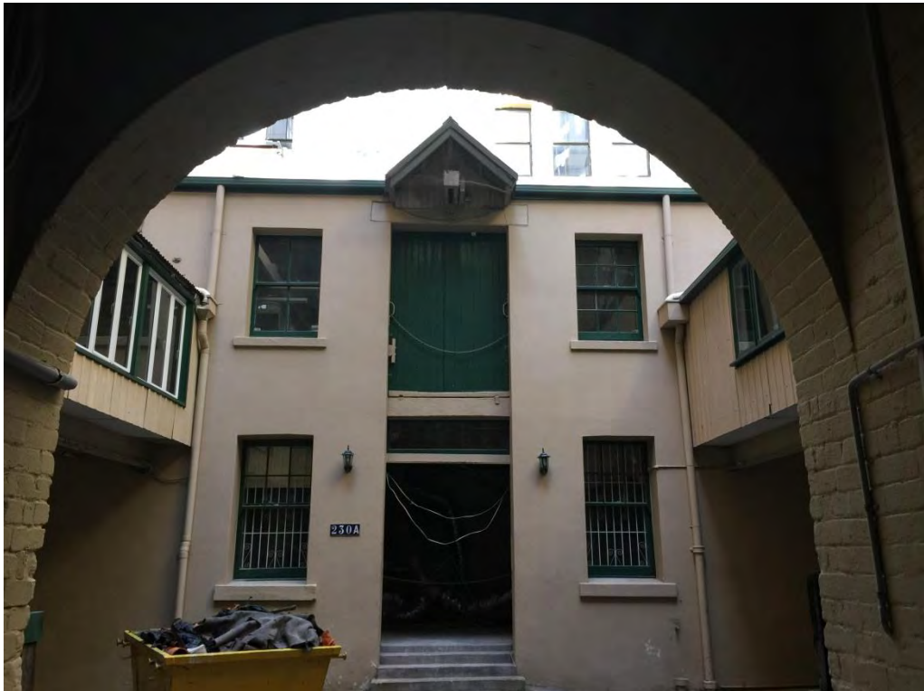
Figure 74 – View through arch of cartway (Y01) western elevation of rear warehouse. NBRS+Partners, April 2015.
