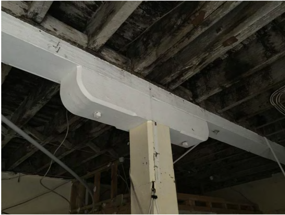
Figure 85 – Beam, bolster and post in space G02. NBRSPartners, April 2015.
