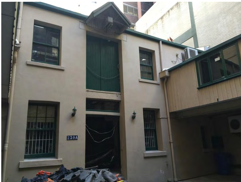
Figure 66 – Western elevation of rear warehouse from yard (Y02). NBRSPartners, April 2015.
