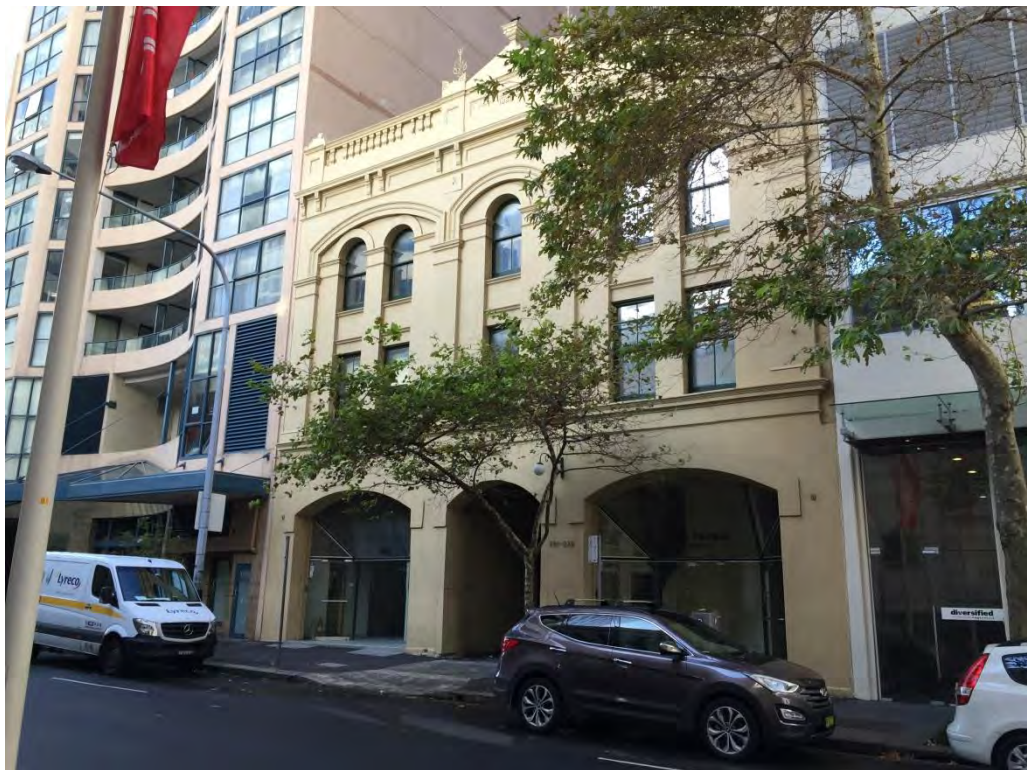
Figure 50 – View to façade from south-west. NBRSPartners, April 2015.
