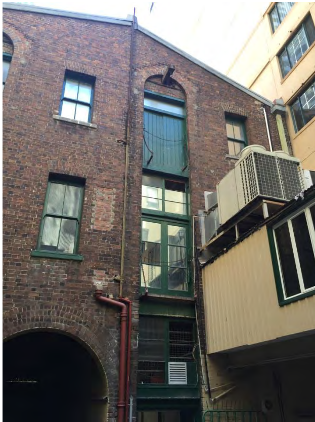
Figure 63 – Eastern elevation of warehouse. NBRSPartners, April 2015.
