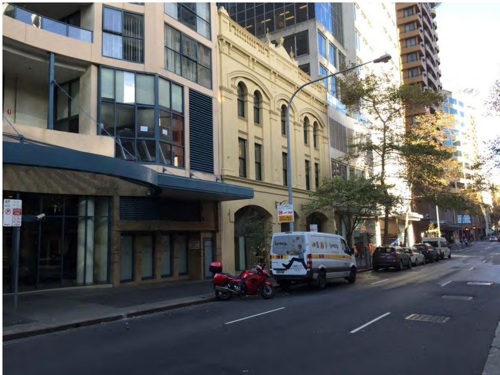
Figure 52 – View to façade from north-west. NBRSPartners, April 2015.
