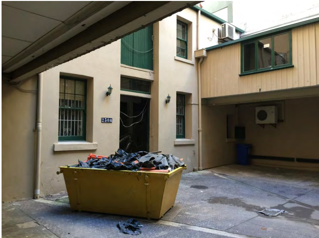
Figure 82 – Yard (Y02). NBRSPartners, April 2015.
