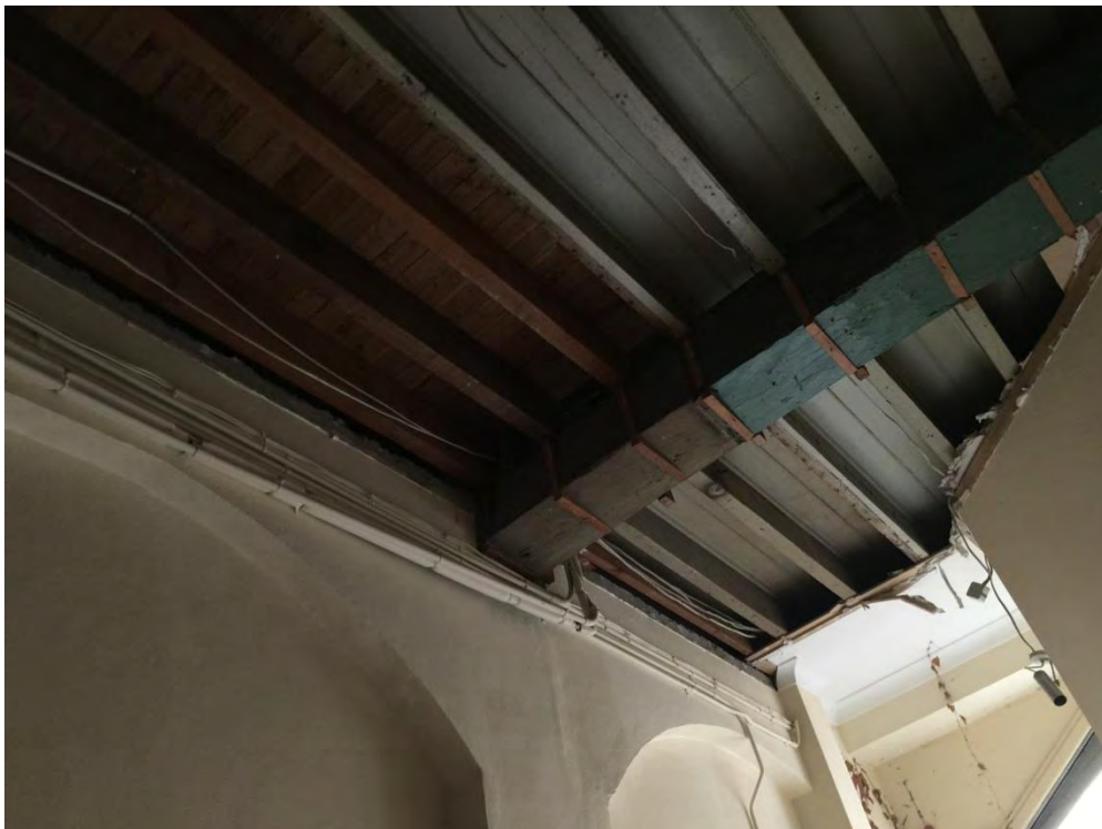
Figure 90 – South-western corner of space G06 showing original matchboard lining. NBRSPartners, April 2015.
