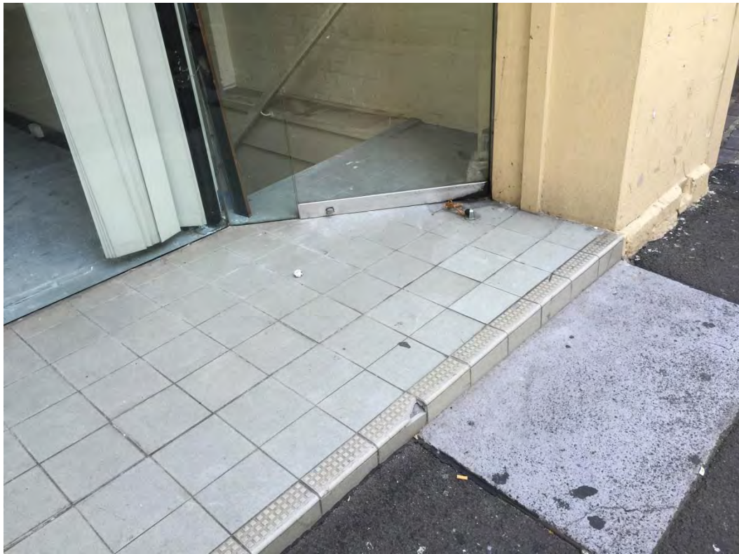
Figure 55 – Altered threshold to infill openings of ground floor. NBRSPartners, April 2015.
