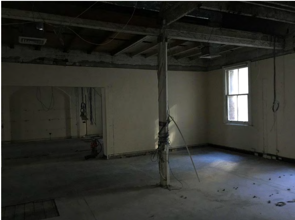
Figure 96 – Eastern section of space S02. NBRSPartners, April 2015.
