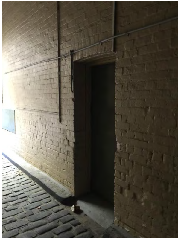
Figure 76 – Former opening in wall to cartway (Y01). NBRSPartners, April 2015.
