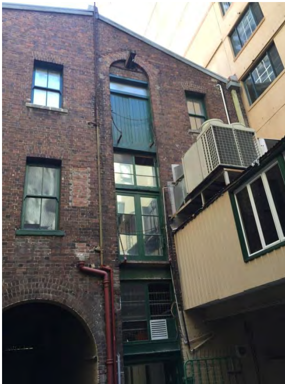
Figure 59 – Eastern elevation of warehouse. NBRSPartners, April 2015.
