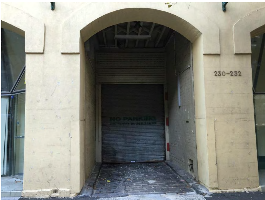
Figure 48 – Entrance to cartway from Sussex Street. NBRSPartners, April 2015.
